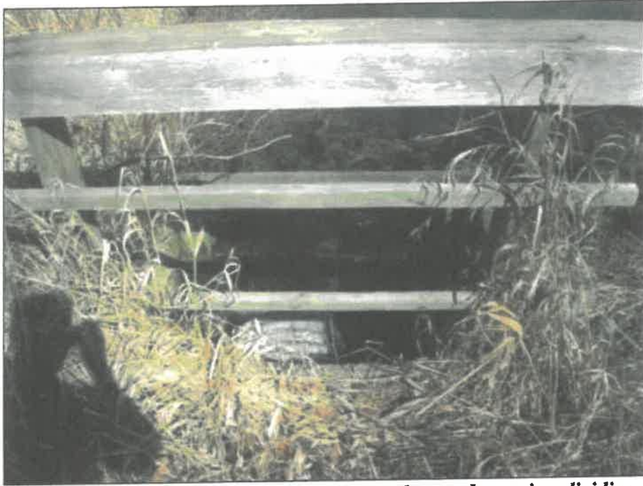
Above: Vertical standpipe allowing flow to pass under road crossing dividing Wetland A and Wetland AA
